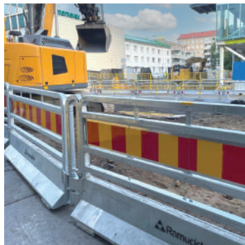
Torun Site Containment Setup
