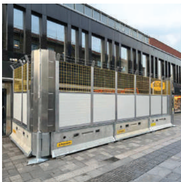
SVEA Complete Site Containment Setup
